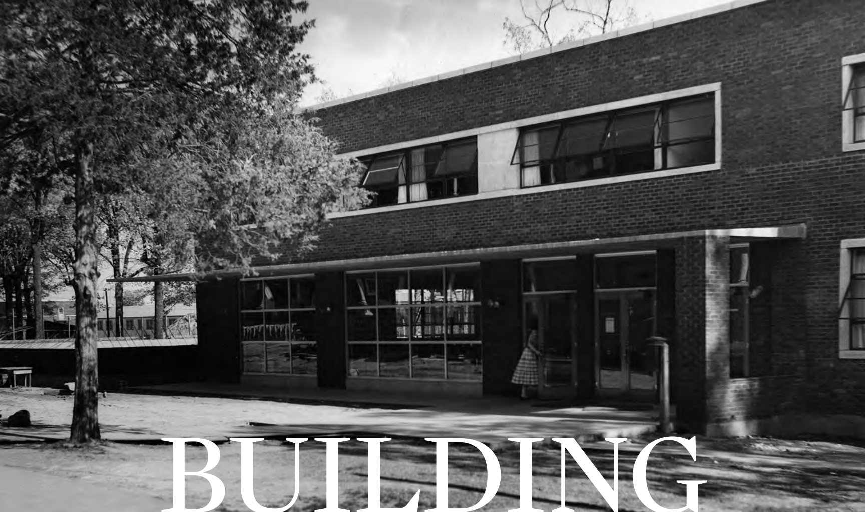
← The Ganus Building first opened its doors in 1951. ↓ Shown in 2017, the Ganus Building is being torn down this summer.
