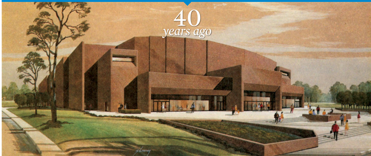
Dedicated March 27, 1980, this rendering was used on the cover of the dedicatory program of Benson Auditorium, which began construction in March 1978. According to the program, "It is a building for the '80s. The strong graphic lines of the new George S. Benson Auditorium reflect a growing and progressive period of campus history. Generous use of space, repeated lighting pattern and semicircular seating combine functionality with the aesthetic." The architect was Yearwood and Johnson of Nashville, Tennessee, and the 58,000 square-foot facility cost approximately $2.6 million and used an estimated 350,000 red bricks.
